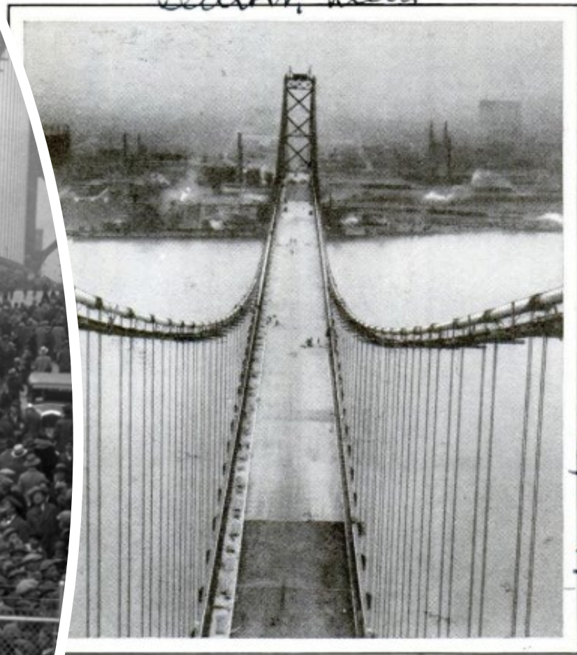
150-Foot Free Span of the "Good Will" Bridge between Canada and the United States, the World's Longest Suspension Span
